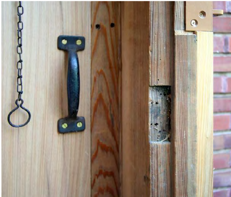
Latch position from mistake.
