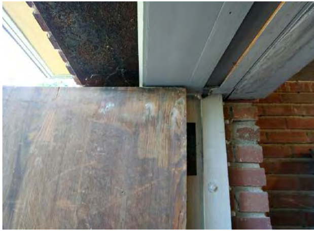
Ghost of mistaken hinge placement.
