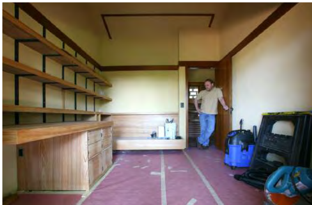
Shelves are supported by welded metal brackets.
