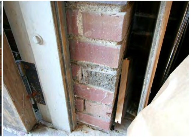
Mismatched bricks where hinges formerly mounted to wall.
