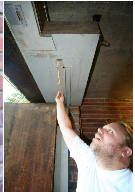
Door stop was improvised from Willey House indoor base shoe.
