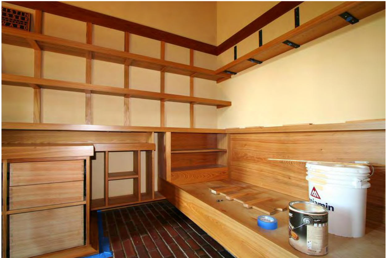
Showing all shelves in place waiting for doors and drawer fronts.
