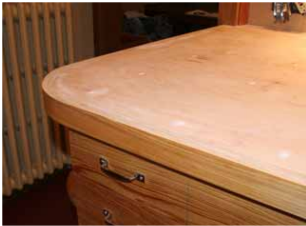
Countertop prepped for the application of linoleum.
