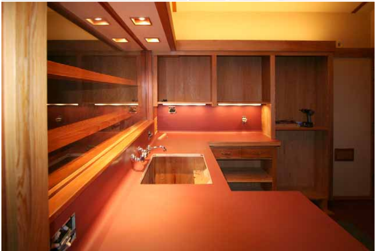
New, single piece linoleum in place.
