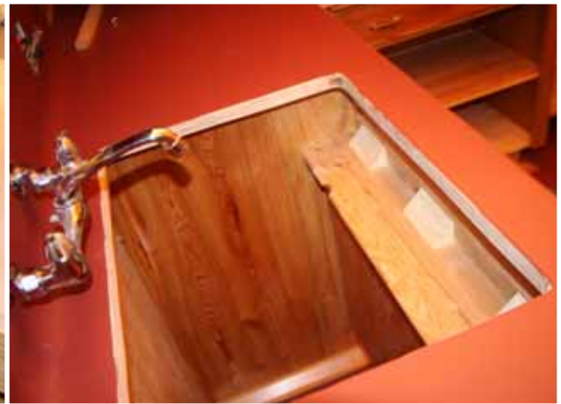
Opening for sink showing wooden supports.
