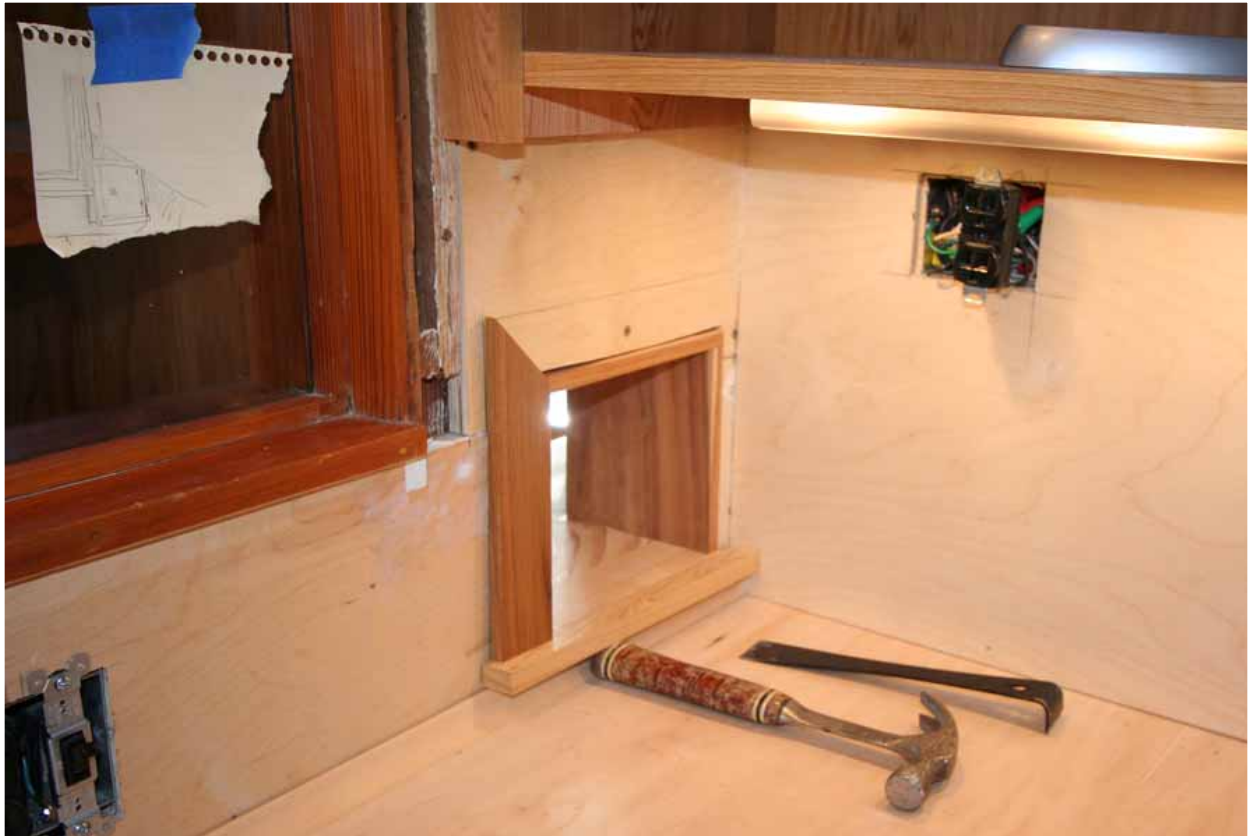
Pass-through being trimmed out.
