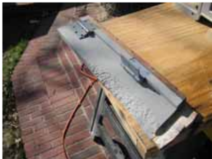
Damaged sill.
