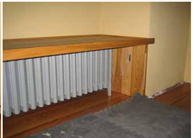
Window seat radiator cover fits into alcove. Faceplate not yet in place.
