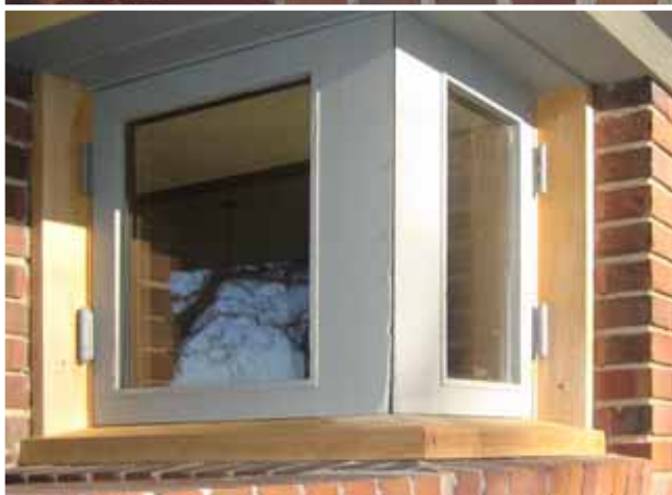
New window sill and frame.
