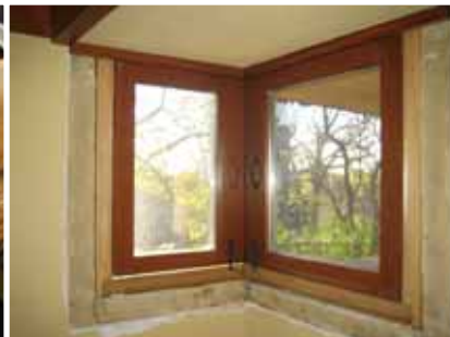
New window sill and frame from inside bedroom. Note original wall color under the interior trim.
