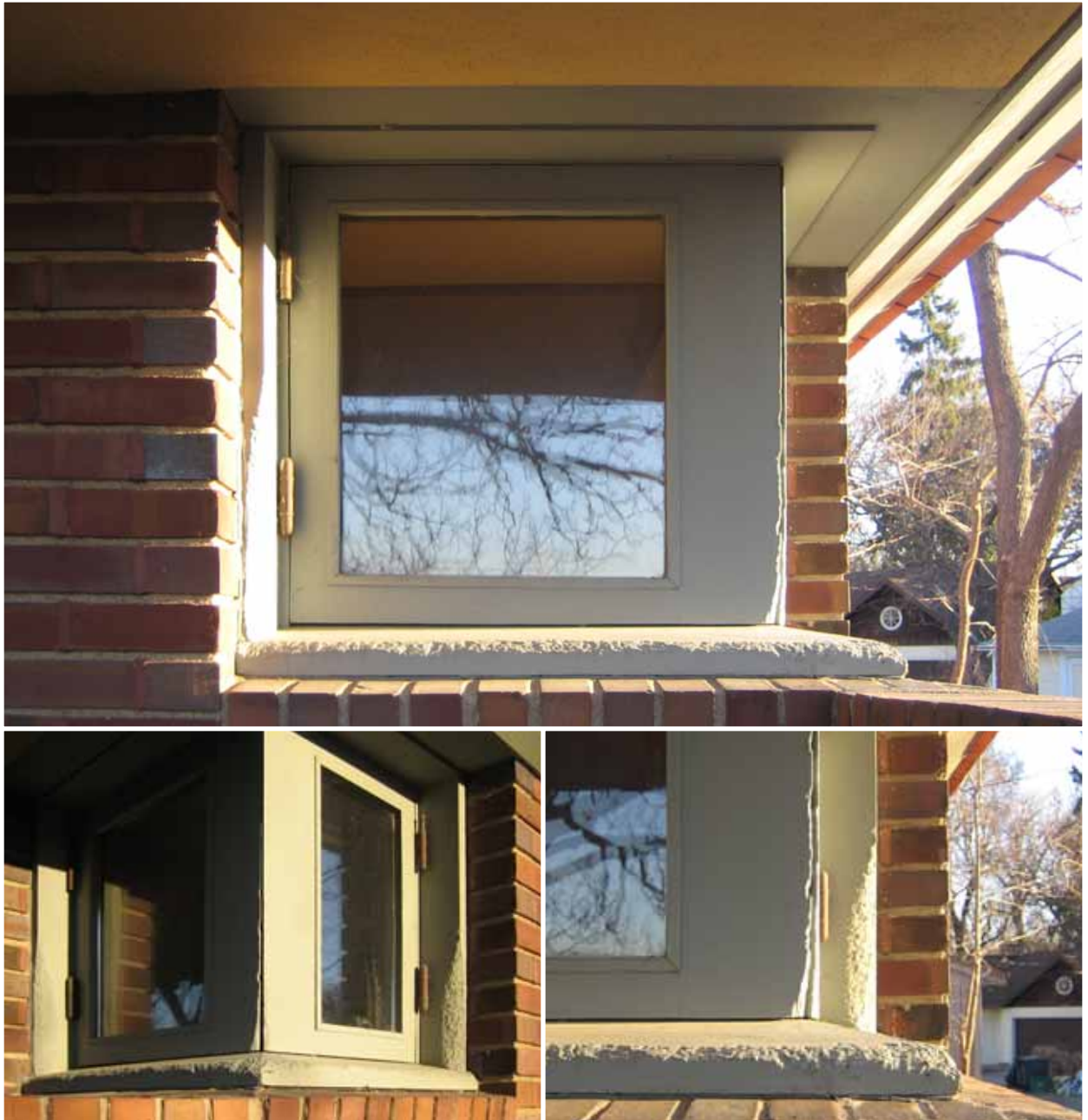
Squirrel-damaged corner window prior to replacement.
