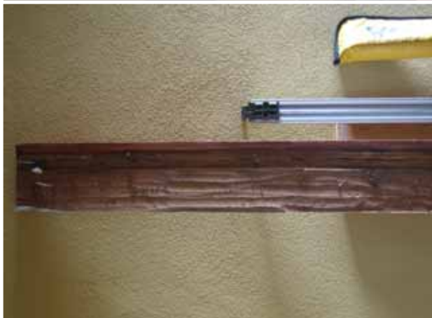
Original sill was hand hewn at the back to fit.
