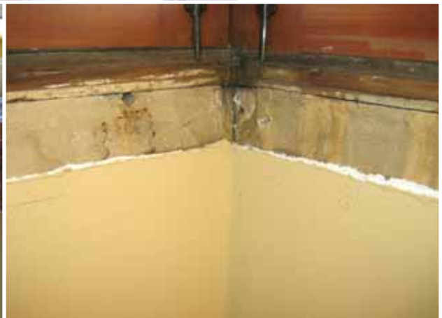
Historic record of leakage, new paint, old paint and tinted plaster.
