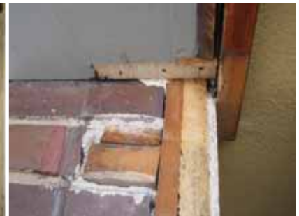
With frame removed the wall structure is revealed. From inside: paint, colored plaster, scratch coat plaster, fiberboard, furring strip, brick and nailer block, stain on exterior brick showing where the window frame ends.
