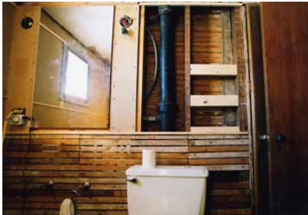
South bathroom wall stripped of plaster.
