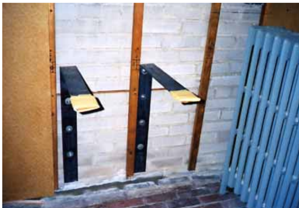
Steel support brackets for the cantilevered vanity table.
