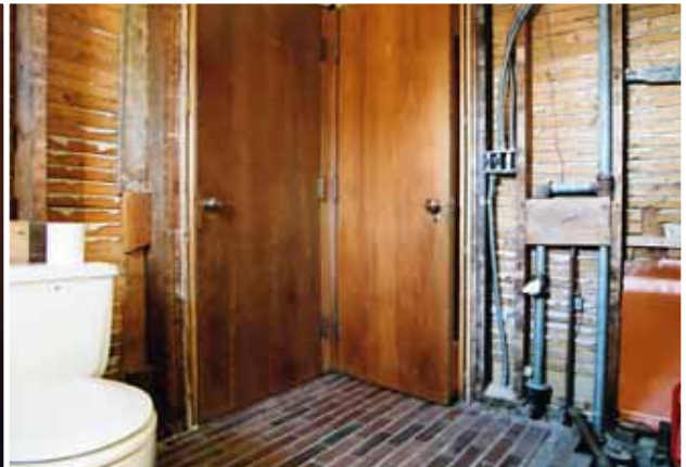
West bathroom wall. Note plumbing for small sink next to tub on the right side of the photo.
