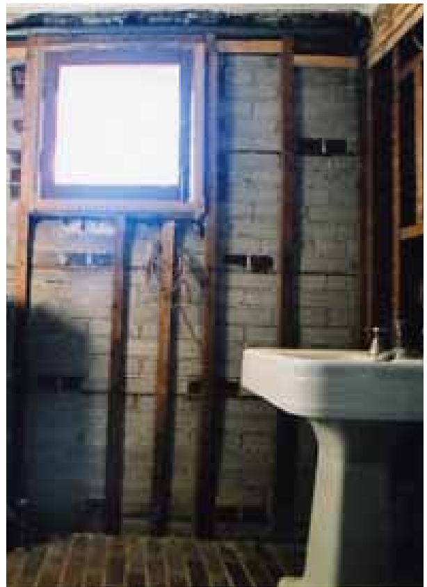
East bathroom wall. Notice the use of cement brick hidden inside the wall, punctuated by red tie bricks.
