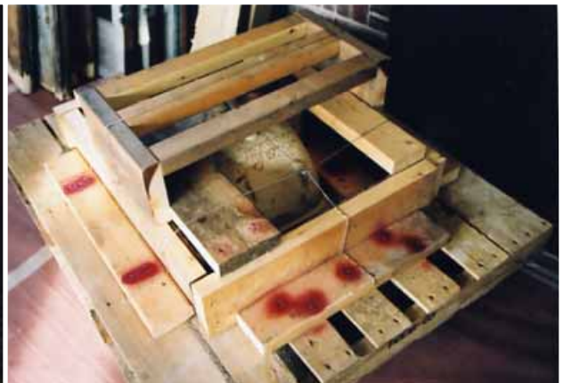
Sink top crated to send off for recoating with porcelain. It is made of cast iron but the porcelain was chipped and worn through. The Bathtub, in a similar condition and was sent to be reporelained also.
