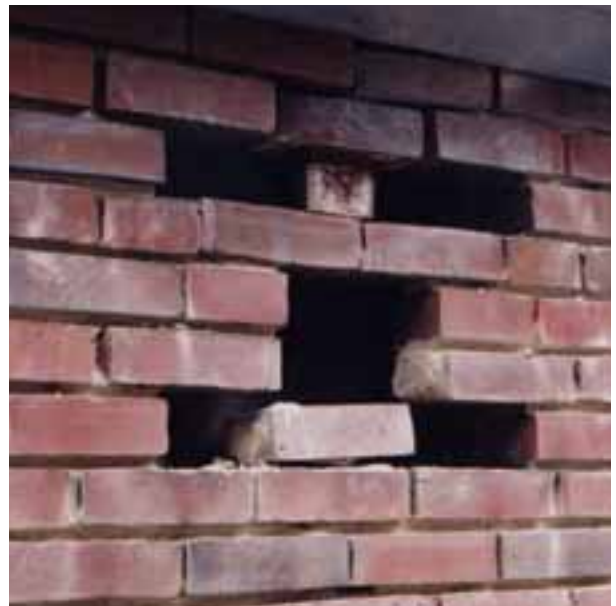
Deteriorated gallery brick screen.
