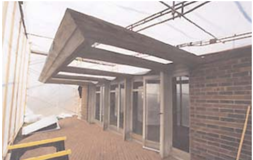
Inside the scaffold tent structure.
